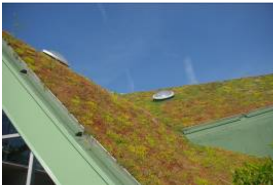
File name: DSC_009.jpg Source: ZinCo / Van der Tol
